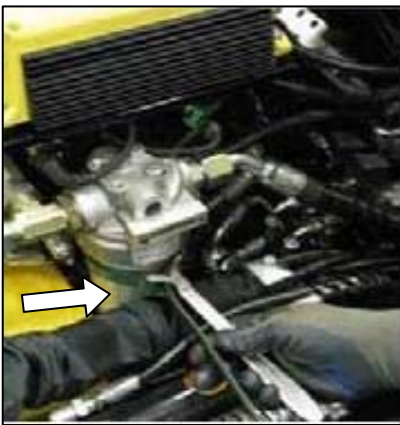
◀ Hydraulic oil filter location
